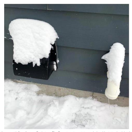
With the recent influx of snow, Saskatoon Fire Department wants to remind residents to check intake pipes and exhaust vents that may be blocked with snow or ice. A plugged exhaust could result in carbon monoxide (CO) being pushed back into your home or cause your furnace to shut down. Residents should check their intake pipes and exhaust vents during and after heavy snowfalls and clear any snow away from the opening if it builds up.
